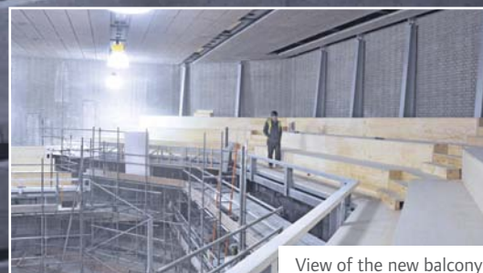
View of the new balcony
