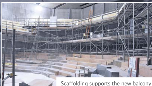
Scaffolding supports the new balcony
